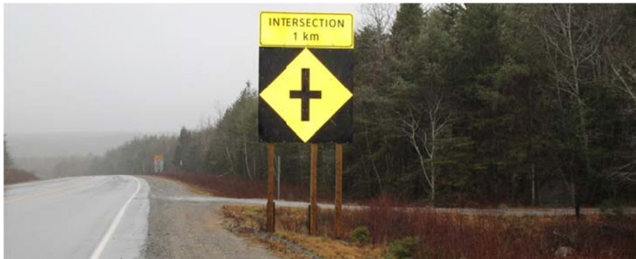
Photo 5-22: While this type of warning sign has been used at some intersections where turns are prohibited, the use of advance warning signs is inconsistent.
