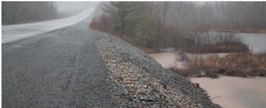
Photo 5-15: This recently repaved or upgraded area with a steep embankment slope near km 206.8 adjacent to a watercourse should be evaluated to determine if guardrail is required.
