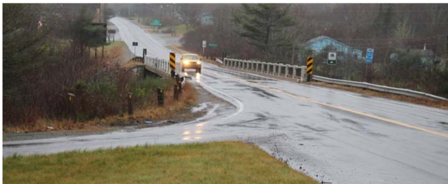
Photo 5-18: The rails on the Jordan River Bridge do not meet the current requirements of the Canadian Highway Bridge Design Code. It is also noted that the approach guardrail does not appear to be fastened to the bridge end.
