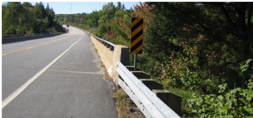
Photo 5-20: This is an example of a typical bridge end treatment. Note that the approach rail has closely spaced and blocked posts with an added steel wheel rub rail, and that the high curb section of the concrete bridge rail is no longer used.
