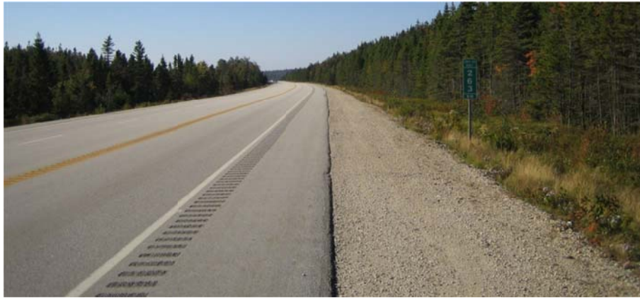
Photo 5-10: Paved and usable shoulder widths at this location appear to meet the Nova Scotia guideline requirements.
