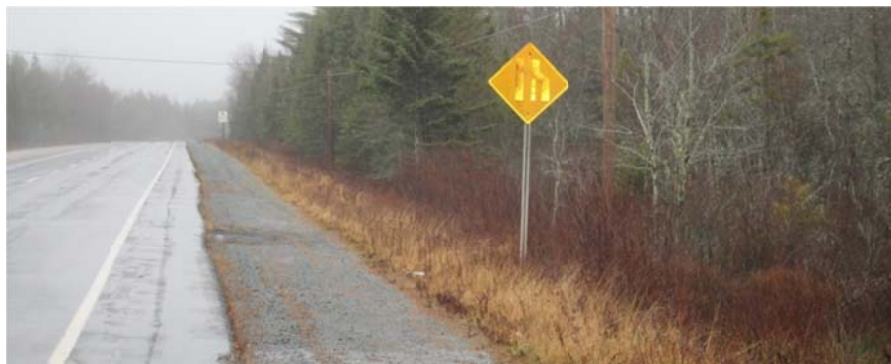
Photo 4-8: This warning zone sign which is worn and faded should be replaced by signage with adequate display and retroreflectivity.
