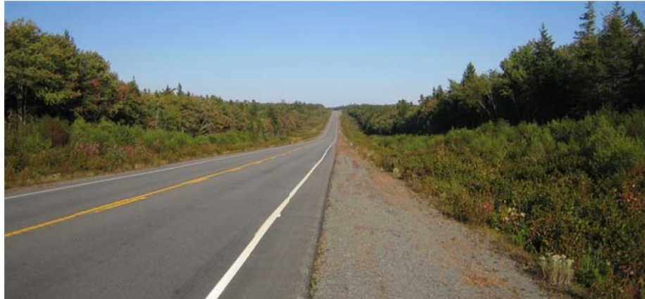
Photo 4-5: While vegetation control appears acceptable, additional cutting will be required soon to keep it from becoming high enough to hide animals.
