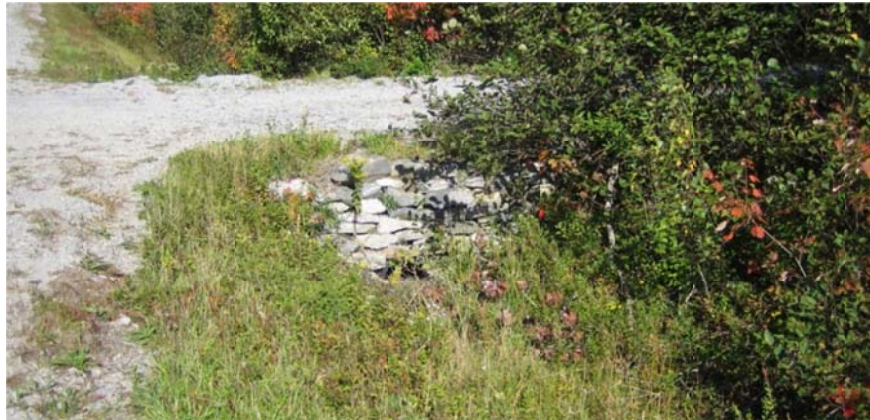
Photo 5-1: Land access and cross median culverts with vertical head walls often have fatal consequences for striking vehicles. Approach slopes should be approximately 10:1 with grates to prevent wheel entrapment.
