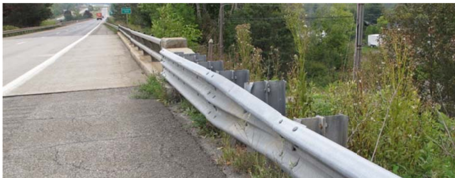
Photo 5-21: This is an example of a typical bridge end treatment used on Interstate 95 in Maine.
