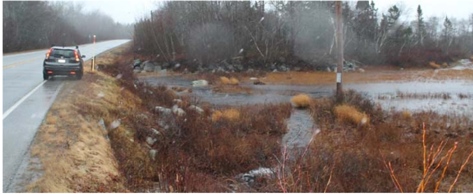
Photo 5-17: This photo illustrates a dangerous and somewhat hidden vertical drop-off at a twin culvert installation at km 123.9. It is recommended that this, and similar locations, installations be adequately protected by appropriate roadside barrier systems, or modified to provide adequate protection for motorists.
