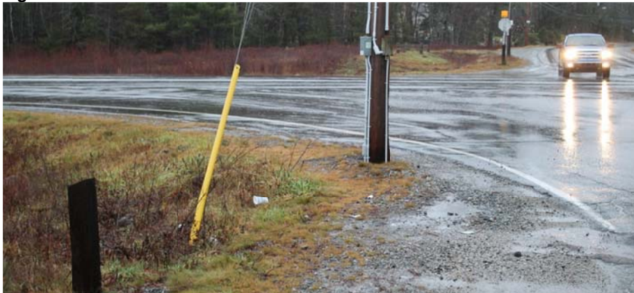
Photo 5-3: This utility pole with multiple services is located at EXIT 26, Ohio Road, Shelburne. While poles are required to support overhead flashing warning lights, they should either be located outside the clear zone, or protected by an appropriate roadside barrier system.
