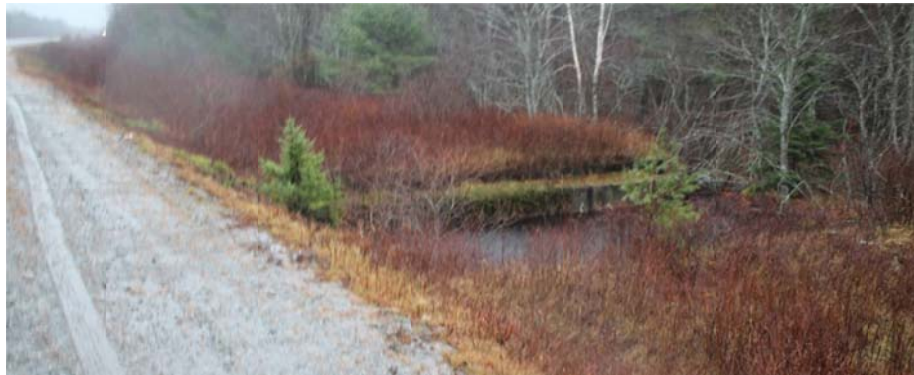
Photo 5-5: This appears to be an abandoned bridge abutment within the roadway recovery area which presents itself as a vertical wall to traffic leaving the roadway. This installation and similar roadside obstacles should either be removed during construction or protected by an appropriate roadside barrier system.
