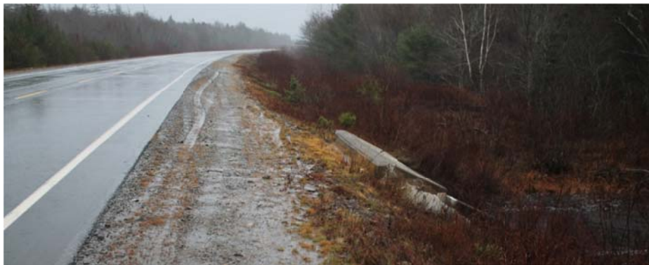
Photo 5-16: Concrete box culverts such as this one at km 105.1, and another one at km 104.5, protrude from the embankment within the clear zone. It is recommended that these installations be adequately protected by appropriate roadside barrier systems, or modified to provide adequate protection for motorists.
