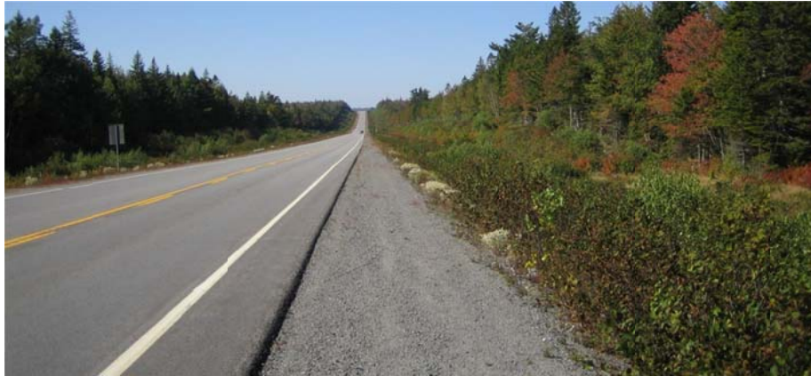
Photo 4-1: The approximately one meter wide paved shoulder does not have a rumble strip.
