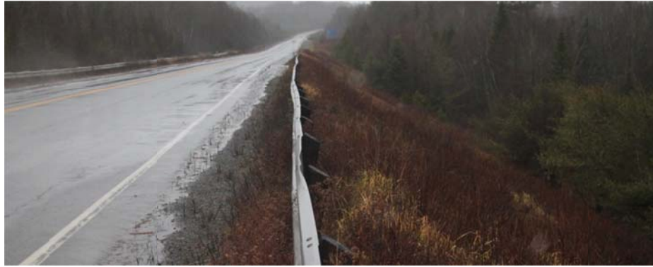
Photo 5-11: This installation includes 3.81 m (12'6") post spacing without blocks. It is also noted that there is only minimal embankment material behind the guardrail to provide lateral earth resistance to the posts.
