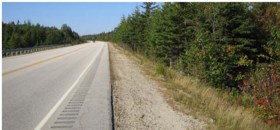
Photo 4-3: Lack of brush control has allowed trees to grow in the ditch area.
