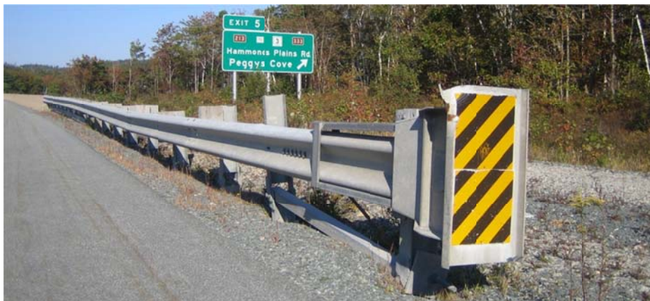
Photo 5-13: This impact attenuating end treatment is similar to the type that should be used on all guardrail end sections on Highway 103.
