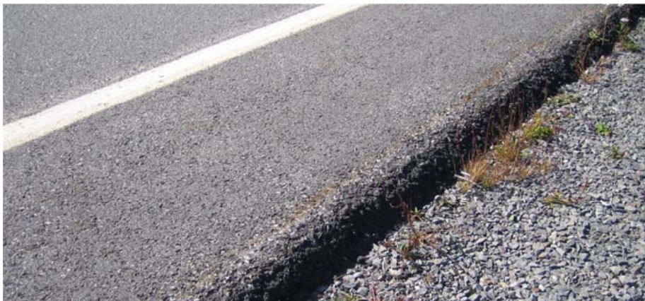
Photo 4-2: The shoulder drop-off appears to be excessive.
