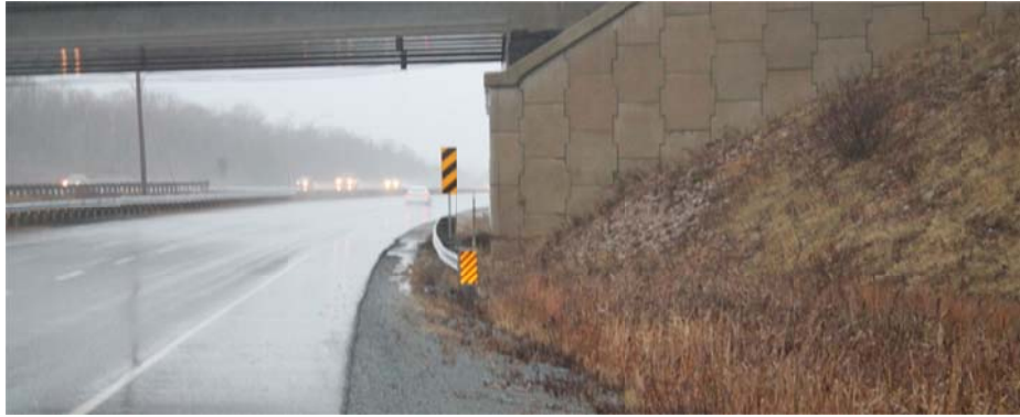
Photo 5-14: While the guardrail end treatment is appropriate, it appears that there is insufficient barrier approach length to adequately protect drivers from the roadside obstacle. It is recommended that barrier approach lengths be reviewed on Highway 103 installations to confirm that there is sufficient length to adequately protect motorists from a hazard.
