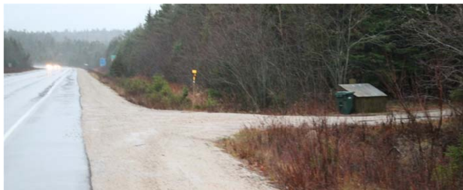
Photo 5-23: This photo is typical of a driveway access directly onto a 100 km/h controlled access section of Highway 103. Since motorists travelling on the highway of this classification do not expect driveway accesses, these locations are potentially hazardous for both highway and driveway users.
