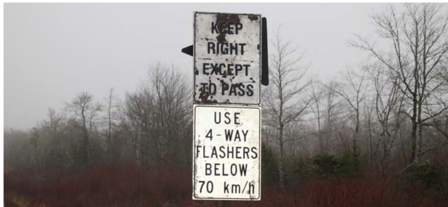
Photo 4-7: This sign, which is worn and faded, should be replaced by signage with adequate display and retroreflectivity.
