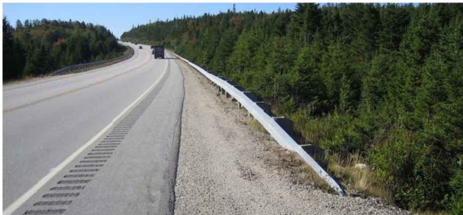
Photo 5-12: While this location has a buried end treatment that may cause a striking vehicle to become airborne, the section beyond the end treatment includes 1.905 m (6'3") post spacing with blocks. This type of end treatment should not be used on freeway or major arterial roadways.
