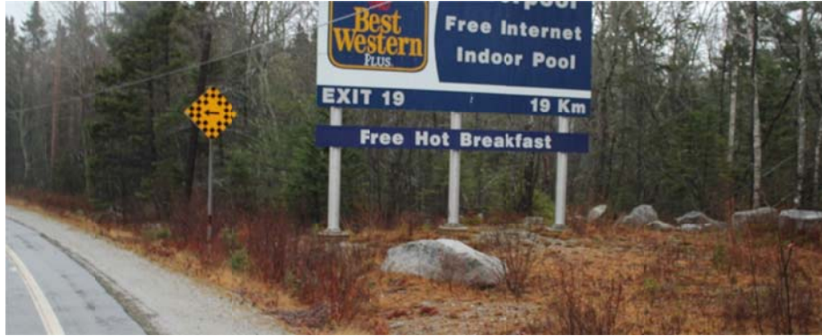
Photo 5-4: The large sign and protruding rock are located approximately seven meters from the edge of pavement. Rock outcrops should be removed during construction; signs should either be located further from the road or protected by an appropriate roadside barrier system.
