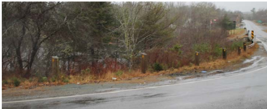
Photo 4-9: The guideposts illustrated should not be used on this road class. The steep embankment appears to warrant a guardrail installation.
