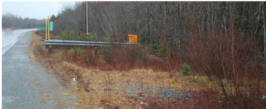
Photo 5-6: This is a utility cabinet that contains an NSTIR permanent traffic counter with guard rail perpendicular to the roadway. If protection is considered to be needed, an appropriate roadside barrier system should be installed parallel to the roadway
