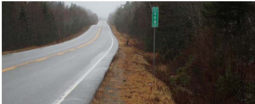
Photo 5-7: Between Sable River and Broad River the paved and usable shoulder widths are significantly less than required by design guidelines. While the completion of the Port Joli and Port Mouton By-Passes will replace a portion of this section with current standard roadways, the remaining parts will still have narrow shoulders.
