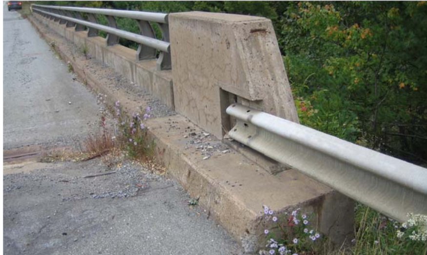
Photo 5-19: This is an example of the older style bridge end treatment where the single bolt is missing. Note that even if a vehicle striking this bridge end did not displace the guardrail and hit the crash block, it would hit the high curved end section of the bridge rail system.
