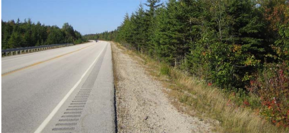
Photo 5-9: While the paved portion is wider than that shown in Photo 5-8, both the paved and usable shoulder widths are less than required by the design guidelines.
