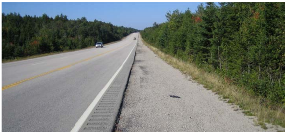
Photo 5-8: This section of highway has a reasonable usable shoulder width; however, the narrow paved shoulder presents a potential hazard for vehicles that may 'hit' the shoulder pavement drop-off. Current guideline width paved shoulders should be provided.
