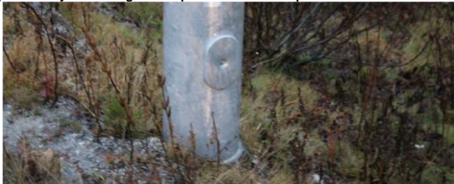
Photo 5-2: Light standards with non-frangible bases become roadside hazards when located in the clear zone. Installations at intersections and exit ramps should use frangible bases.
